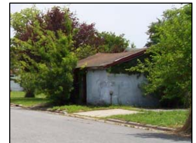
Image of dilapidated structure on Hammond Street near a school
